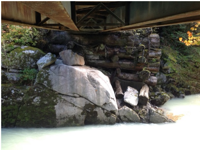
Left Bank Abutment when facing downstream
