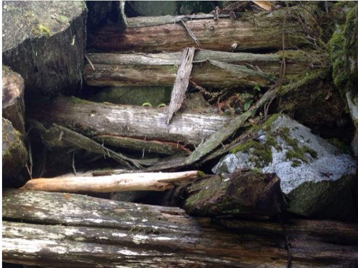
left downstream wing wall
