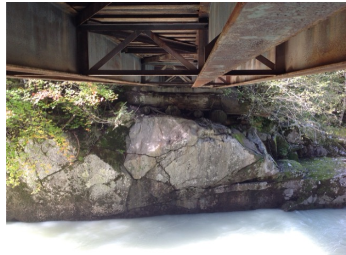
Right Bank Abutment when facing downstream
